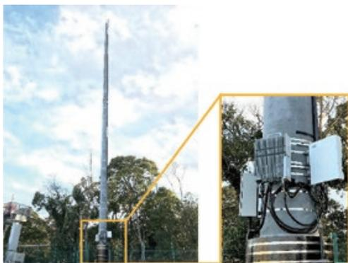
Private BWA base station with 30-meter antenna mast and wireless station terminal at the Chiba Plant
