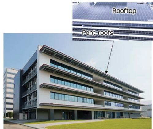
SUSTIE® exterior. Equipped with solar panels only on the rooftop and pent roofs, the test facility shows that ZEB can be deployed even in urban areas with restricted site areas.
